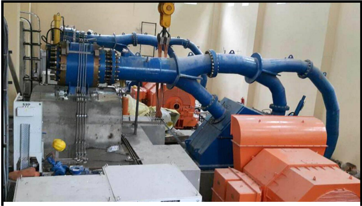
Figure 6.5- 1 3-Jets Horizontal Shaft Pelton Turbine
